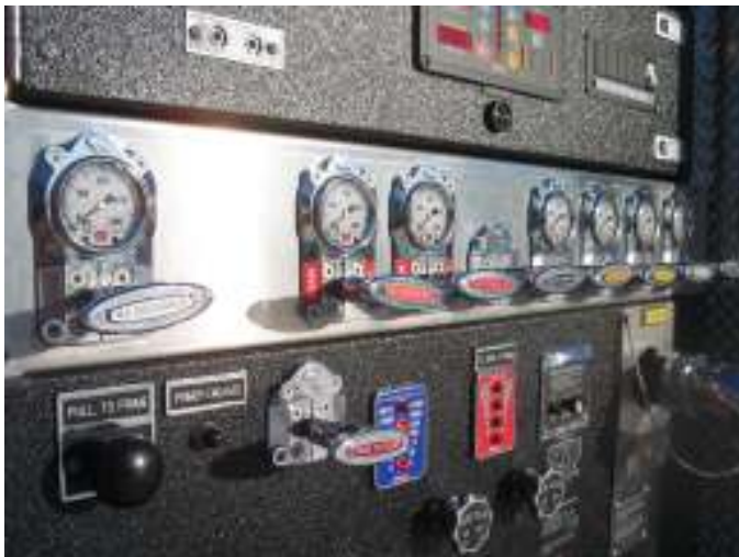
Side Control Fire Pump Panel
